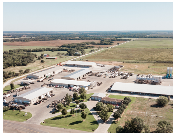
Gore Nitrogen headquarters in Seiling, Oklahoma
